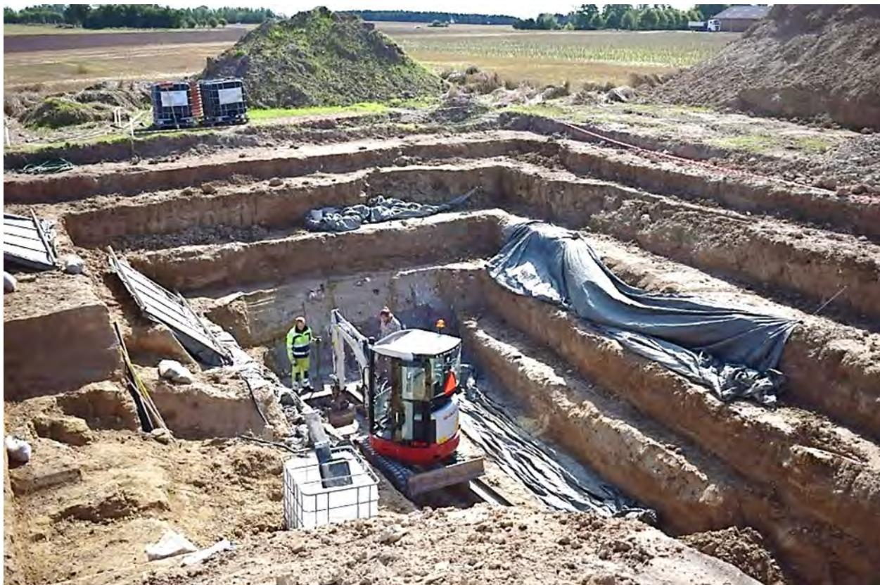
**FIGURE 5.** High-ground excavation E2 in Salløv. Ongoing preparation of the dye infiltration experimental fields BB5 and BB6 in the bottom of the excavation (5.2 m depth).
